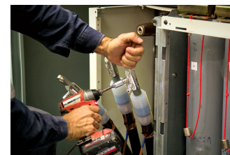
Fig.3 Shear off bolts
